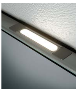
Detail of emergency light
